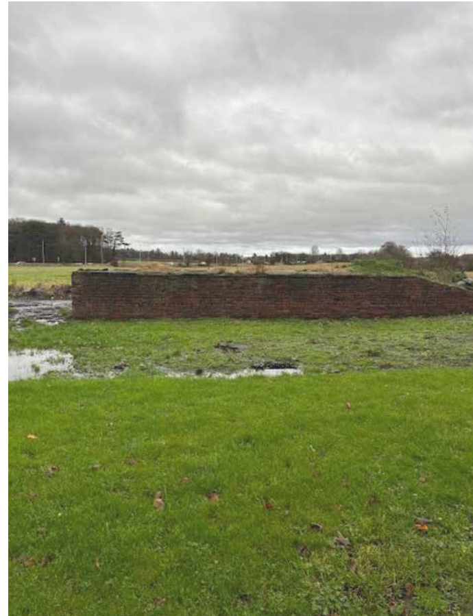
The existing structure
